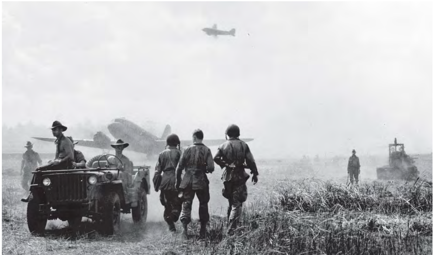
Engineers labor to make the airstrip at Nadzab operational. One C-47 transport has already landed while a second plane appears to be circling or preparing to make its approach to the field.
